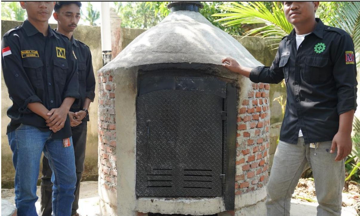
Figure 6. Engineering-Based Combustion Technology Installed for the Community Empowerment Program.
