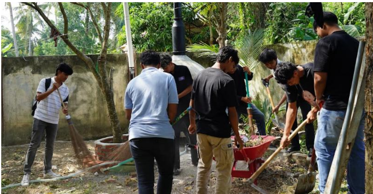
Figure 4. Site Preparation and Cleaning Activities for the Installation of Engineering-Based Technology.
