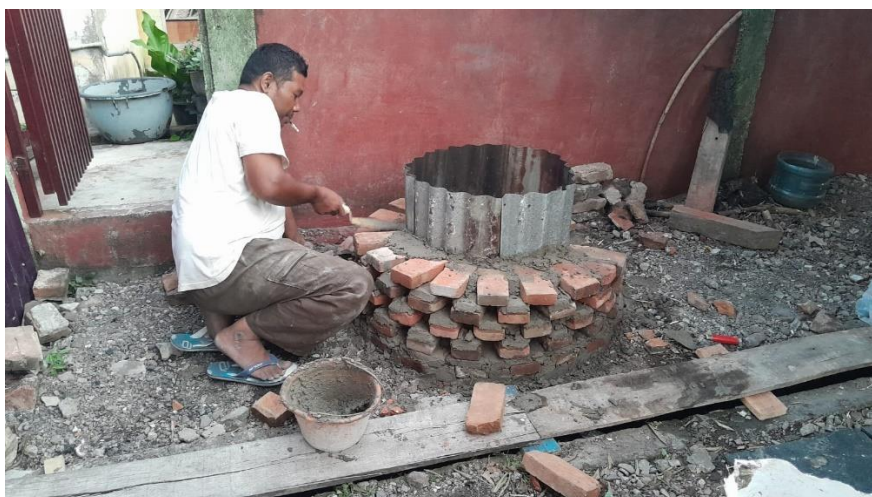
Figure 8: Construction of a Simple Community Waste Incinerator
