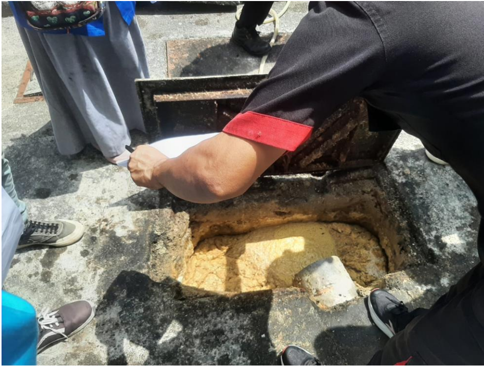
Figure 7: Inspection of the Grease Trap System by the Partner Representative during Field Assessment
