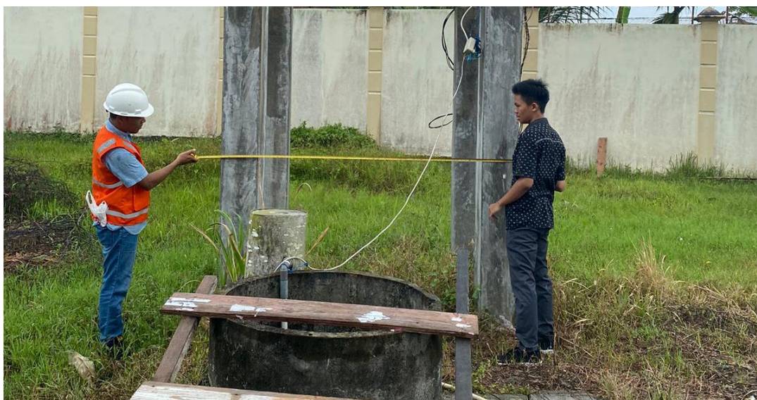
Figure 6: Measurement and Preparation of Water Pump Installation for Solar-Powered Irrigation System
